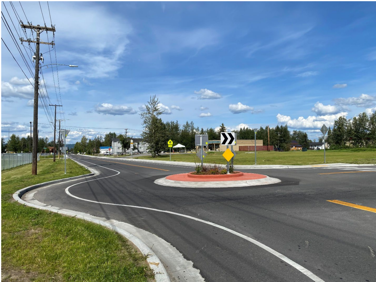
Figure 22: Traffic Circle on Gillam Way in Fairbanks
