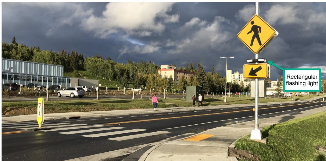
Figure 19: Electrical Warning Devices (Rectangular Rapid Flashing Beacon, or RRFB) on University of Alaska Fairbanks Campus
