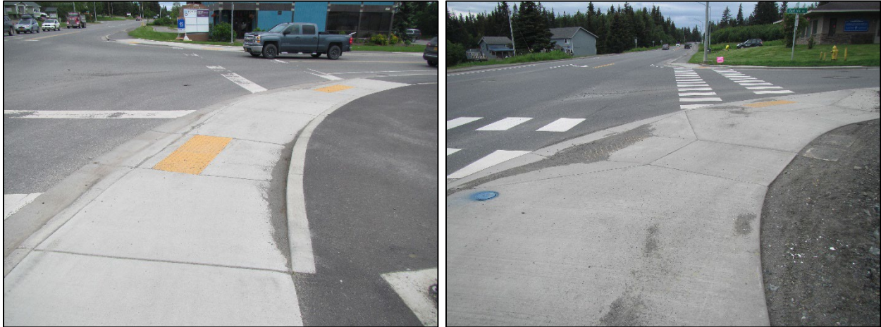
Figure 16: Curb Ramps that Direct the User into the Crosswalk
