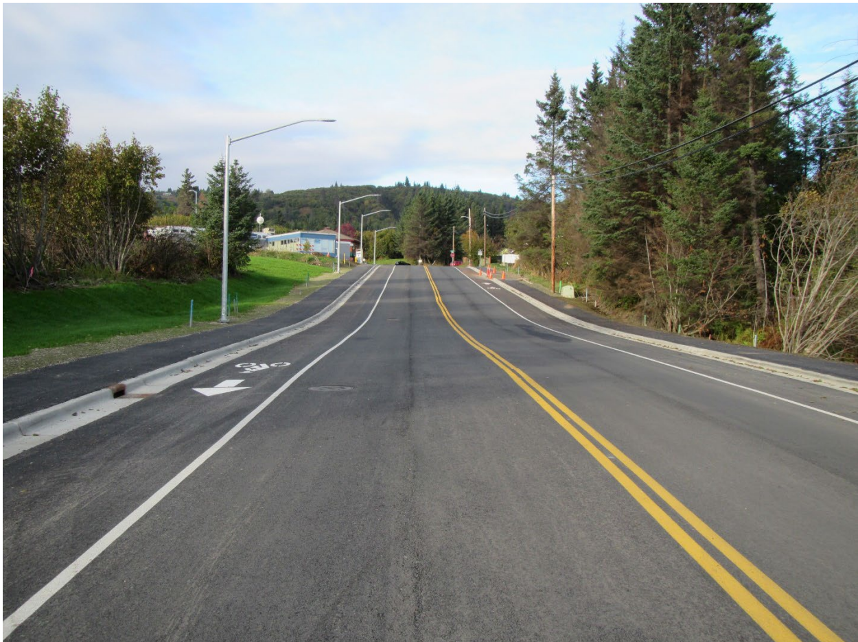
Figure 8: Newly Constructed Greatland Street
