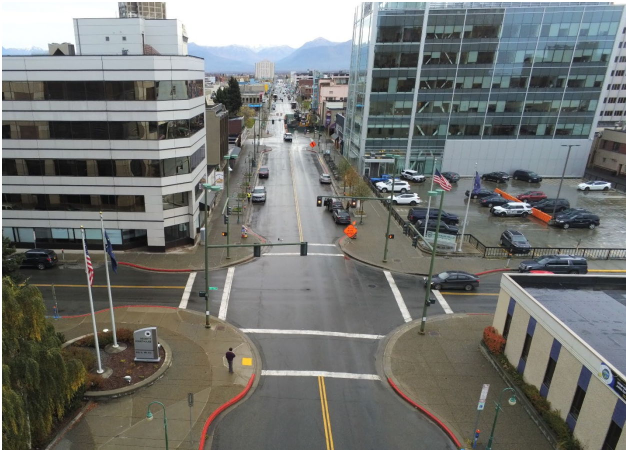
Figure 21: Curb Bulb-outs in Downtown Anchorage, Alaska
