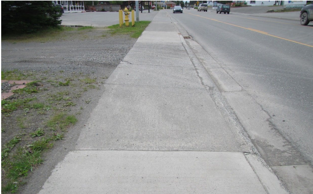
Figure 17: Driveway Entrance with Steep Cross Slope
